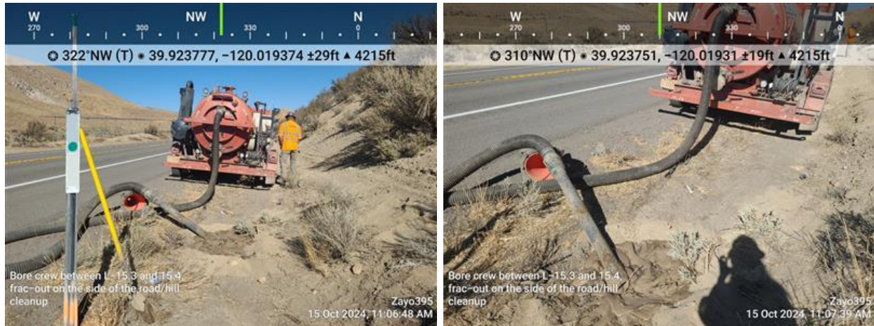
Figure 7. View of frac-out being cleaned up Southern Area (Lassen County).
