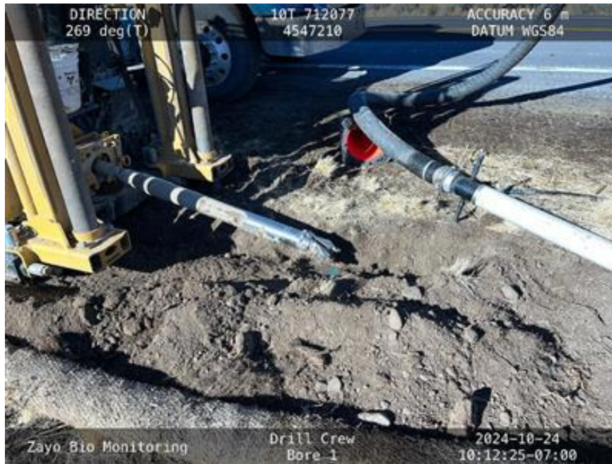
Figure 10. SWPPP Photo - Bore pit with straw waddle and Vac-Truck.
